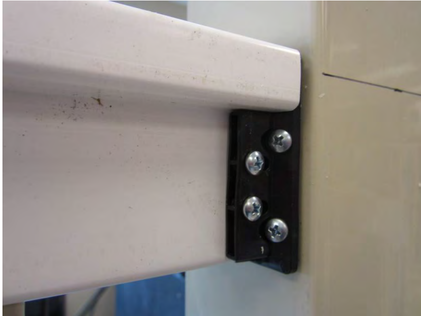
Photo No. 9 "T" Shaped Top Rail-Bracket-Post Attachment
